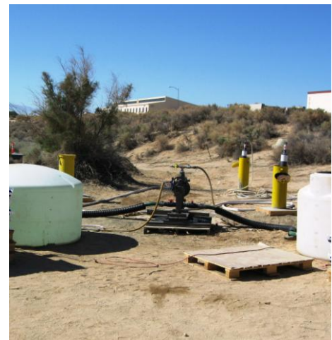
Exhibit 2. Typical ISCO Injection
